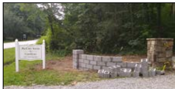
The base for one of the new wing walls takes shape.
