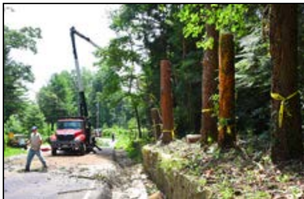
Trees shown with yellow ribbons were first topped, then cut and removed, so that no root disturbance harmed the wall.
