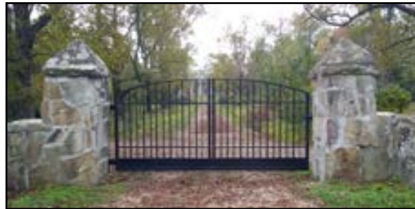
Restored Anderson Pike entrance with coordinating gate
