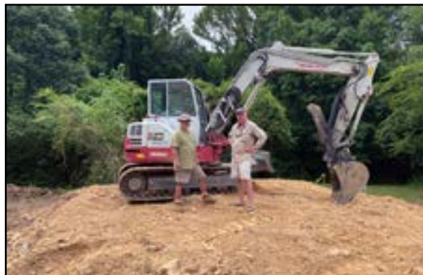
David Clark, builder, and Tom Mills, site preparation.
