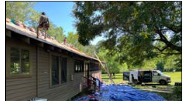
The Pavilion is one of the buildings getting a new roof.
