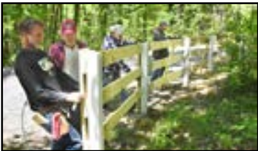
Mark Turner, owner of Middle Valley Fence Company, cuts the tops of the fence posts at an angle so that rain and snow will not pool on top. This method also assures that all fence posts are of equal height. Photo by Charlie Stone.
