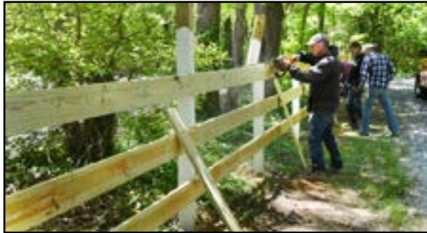
Mark Turner, owner of Middle Valley Fence Company, cuts the tops of the fence posts at an angle so that rain and snow will not pool on top. This method also assures that all fence posts are of equal height. Photo by Charlie Stone.
