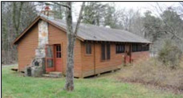
*BEFORE: Unpainted Pavilion with broken chimney and bar-b-cue, door that would not close, "Keep Out" warning, and overgrown Horseshoe Garden. Photo Charlie Stone*
