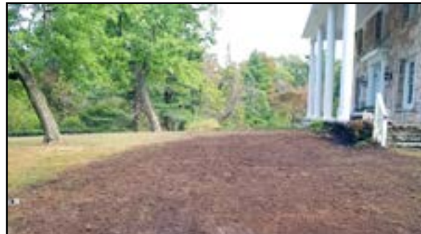
The Big old Silver Maple stump is gone from in front of the house, and the lawn is being prepared for rehabilitation and reseeding. Thank you Grounds Volunteers!
