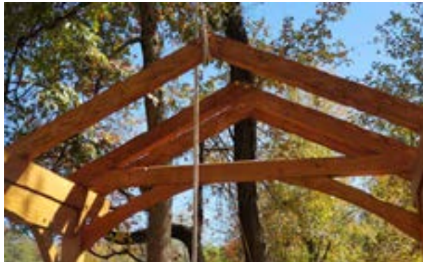
Rafters were raised and placed using a pulley system.
